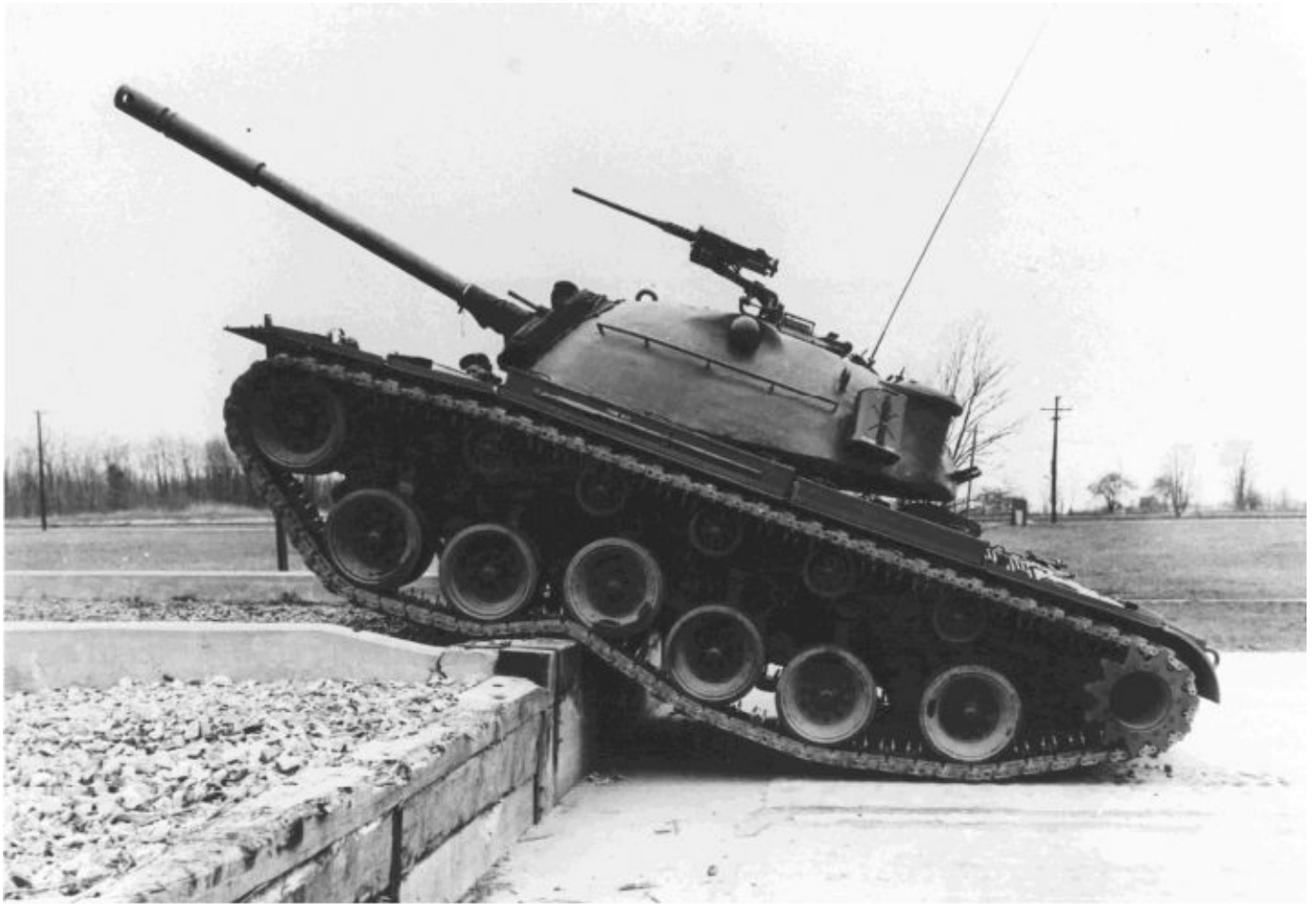
An early model T48 tank climbs over a 36 inch (91.4cm) step at Aberdeen Proving Ground, Maryland, former home of the U.S. Army Ordnance Corps. Testing of the T48 tank revealed that its turret and fire control system did not function properly. The U.S. Army decided to await future turret and fire control developments and continued with production of the vehicle. Patton Museum
