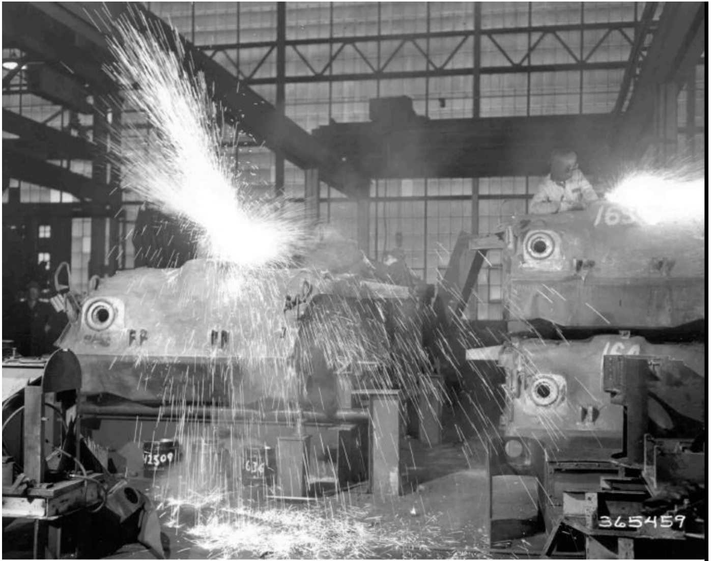
A picture from the production line shows welding being done on the hulls of M46 tanks. The hull of the M46 tank was 20 feet 10 inches (6.36m) long and retained the same armor thickness as the M26 tank series. TACOM
