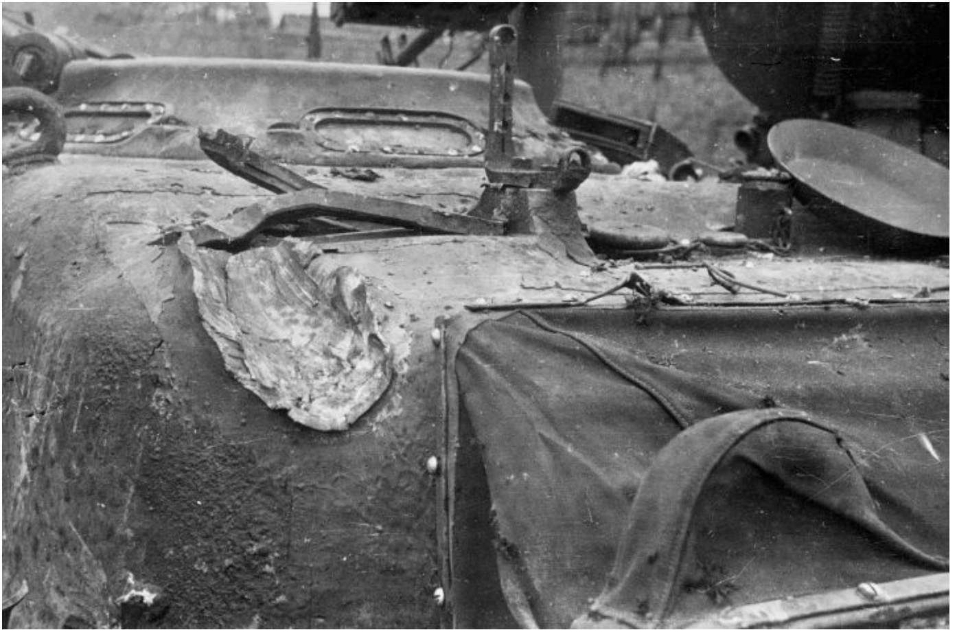
The first U.S. Army T26E3 tank knocked out in combat during the Second World War was serial number 38 and nicknamed "Fireball" by its crew. It took three hits from an 8.8cm gun mounted on a German Army Tiger E heavy tank in late February 1945. Pictured is the third strike on the vehicle that gouged out a chunk of the turret. Patton Museum
