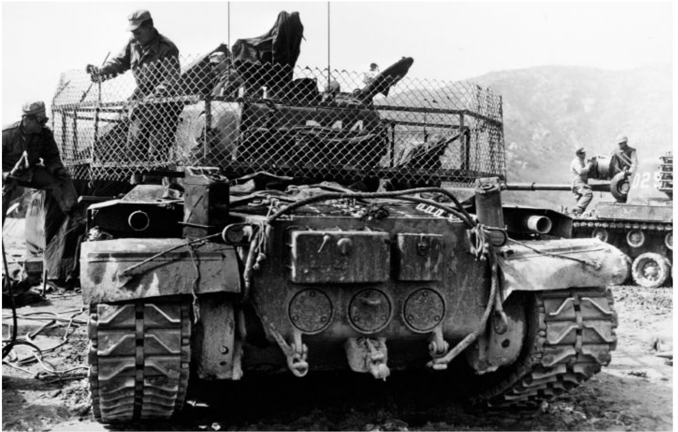
Marines are shown installing heavy wire fencing material around the turret of a M46 tank, sometime during the Korean War. The wire screen was intended to protect the tank from the high explosive antitank (HEAT) warheads of enemy rocket launchers. Notice that the M46 tank has three circular cross-drive transmission access panels instead of the three square ones on the T40 tank. Patton Museum
