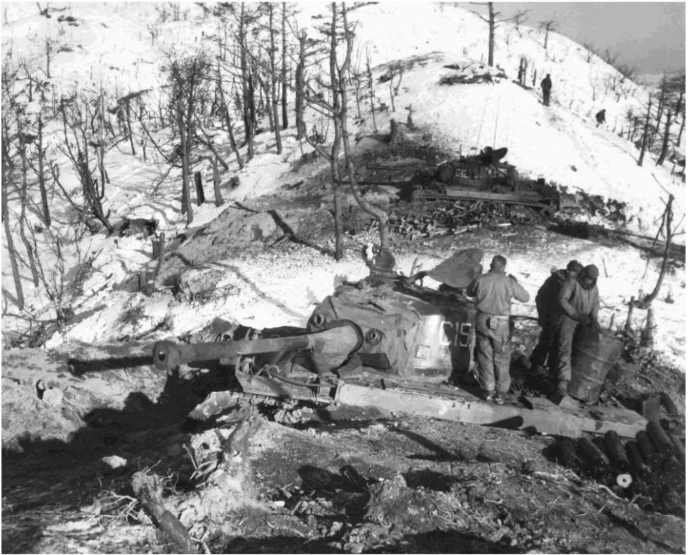
American M46 tanks were often brought to the crest of Korean hills as seen here to provide infantry fire support. The downside of this support activity was the mechanical abuse inflicted on the tanks by continuous climbing of steep hills that resulted in output shafts and final drives failing. Patton Museum
