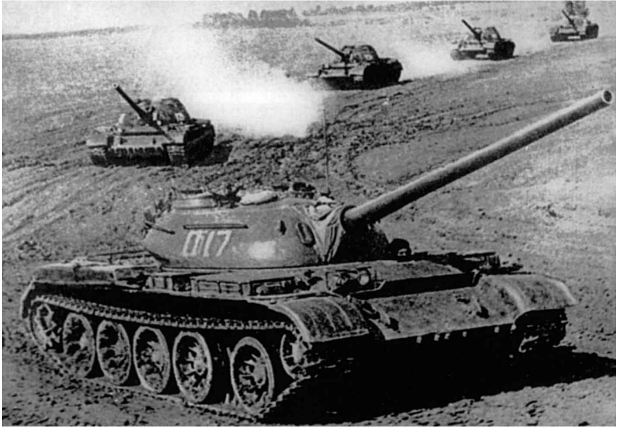
A column of T-54-2s on manoeuvres – the third version of the turret would dispense with the shot trap at the back.
